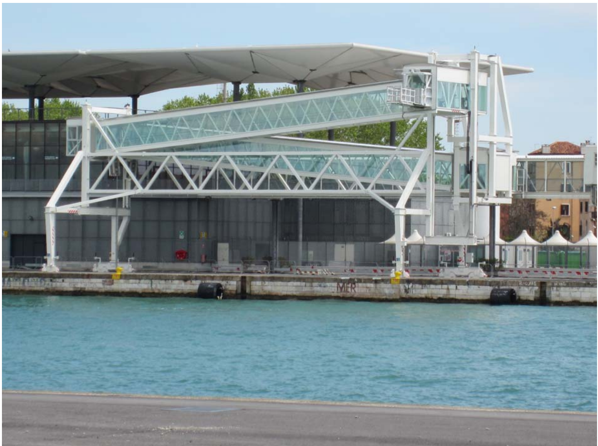
1. S.B.B. ship boarding bridge installata in banchina Isonzo
